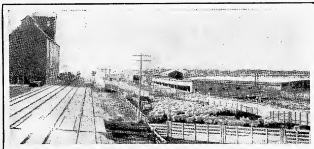
AN ILLINOIS FEEDING AND SHIPPING YARD.
