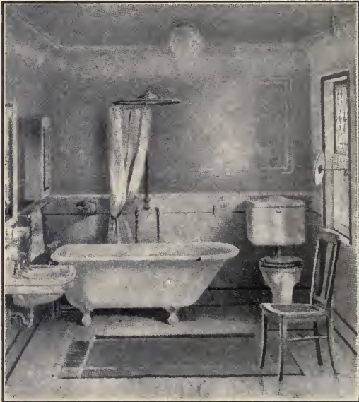
FIG. 16. — A well-fitted bathroom, the fixtures sanitary and simple.
