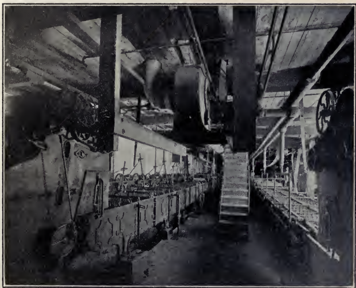
FIG. 66. — Wool washing or scouring. Notice the rakes in the machines which move the wool back and forth in scouring.
