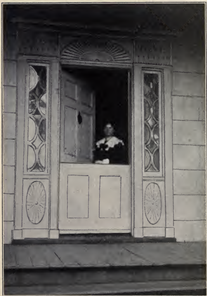
FIG. 12. — A postcolonial doorway, New Jersey, about 1800.
