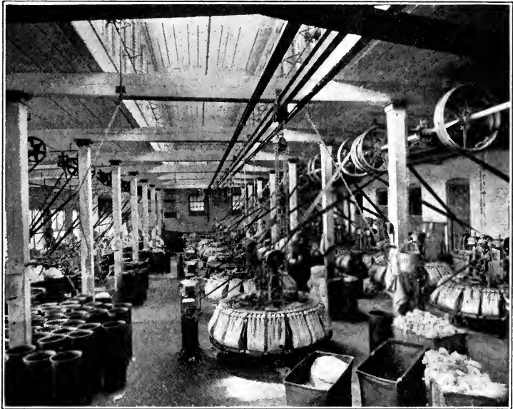
FIG. 68. — Wool combing. This machine is used in the manufacture of high grade wools. There is much waste.
