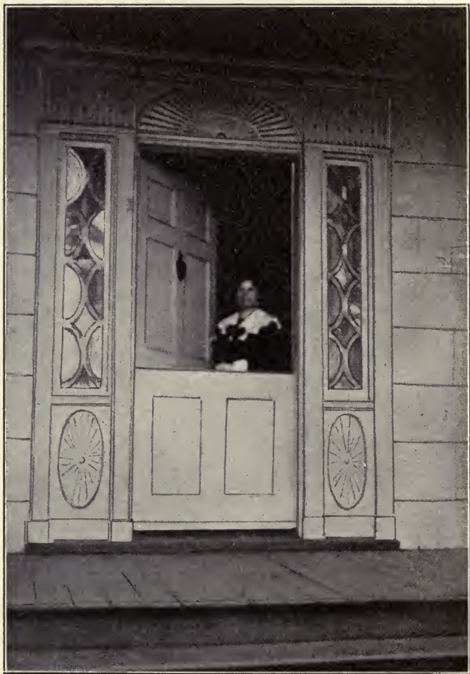
FIG. 12. — A postcolonial doorway, New Jersey, about 1800.
