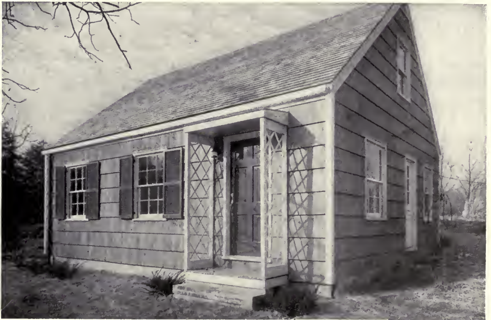
FIG. 6 ( above ). Low-cost housing. Erection of a prefabricated house in sections. FIG. 7 ( below ). The completed house a few hours after work was started. A successful solution.
