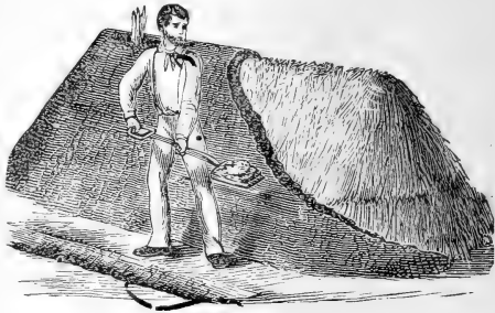
Fig. 1.—PIT FOR ROOTS.
