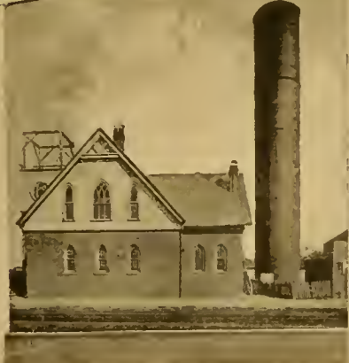
Methodist Church and Water Tower
