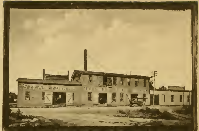
Sherman Iron Works.
