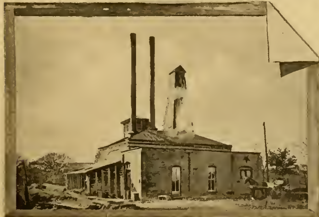
Pumping Station of Water Works
