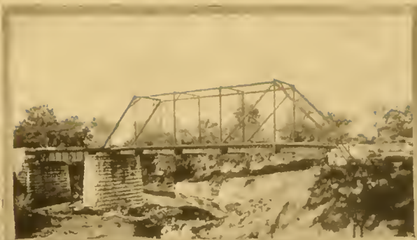
H&T.C. RR Bridge.
