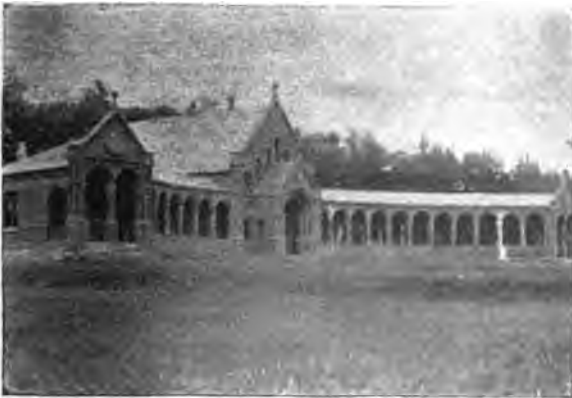
POWERS MEMORIAL BUILDING.
