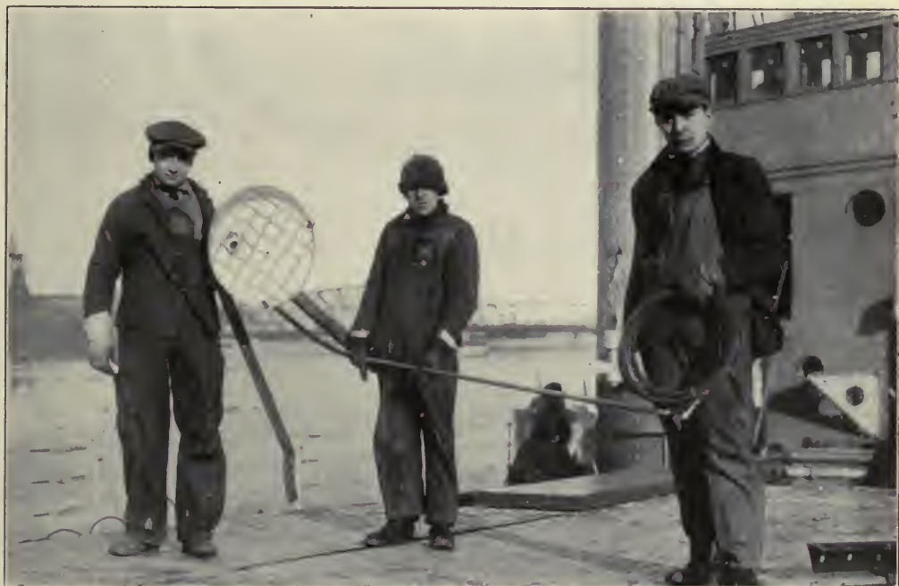
Electricians Installing a Search Light
