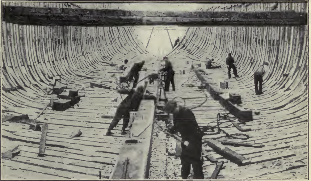
Schooner in the framing stage, showing the laying of the keelson.
