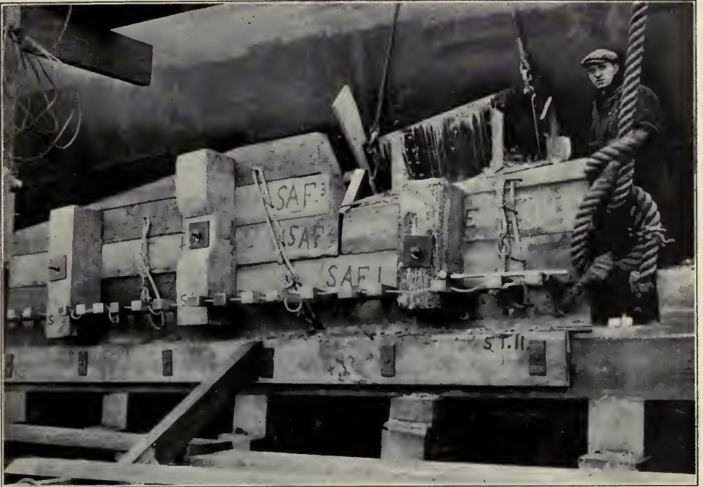
Launching Ways. In launching, the upper part of the ways slides upon the lower, carrying the ship into the water.
