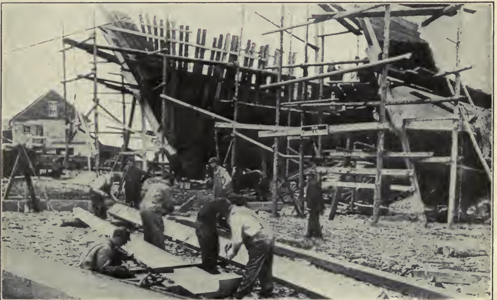
Shipwrights shaping timbers with the adz.
