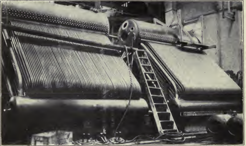
Assembling water tube boilers.
