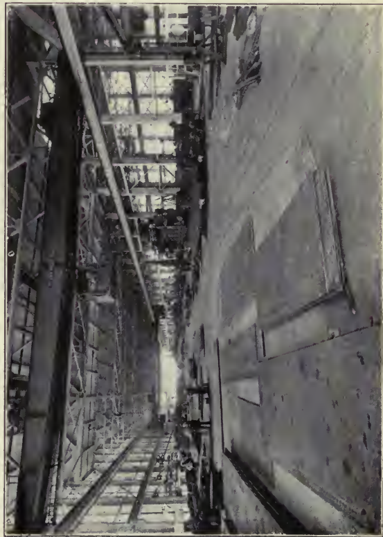
The ground floor is in two divisions. On one side, plates for the hull are
