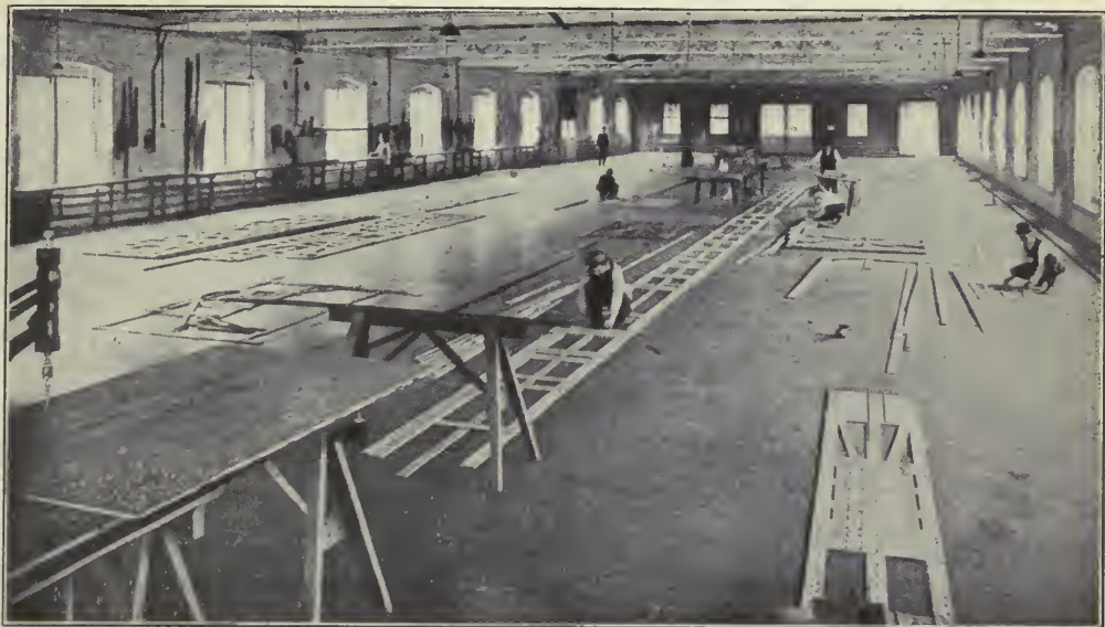
Laying out work preliminary to construction of vessels. (Courtesy of "American Machinist.")
