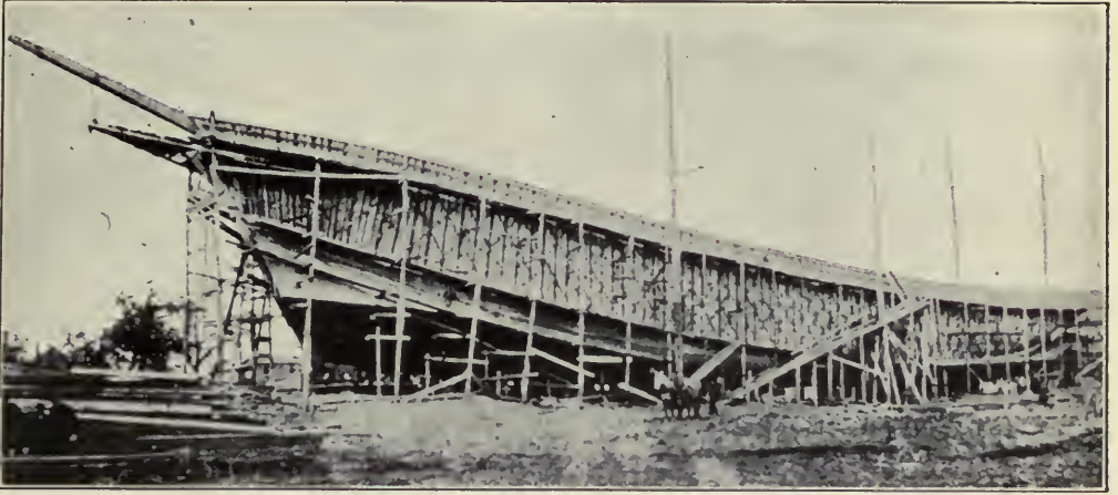
Ship planked just above the water line, showing the ribs of the upper part and the cross pieces of steel used for reinforcement.
