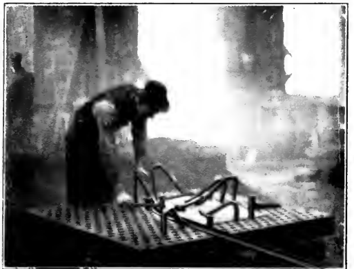
(2) The Anglesmith, bending a small bar into the shape required for use in a ship.
