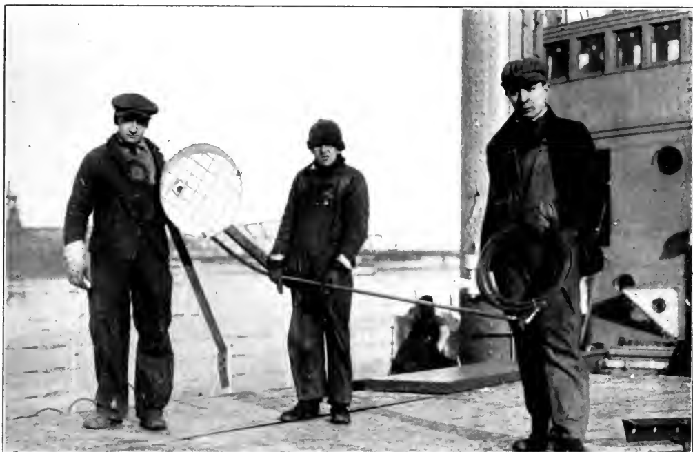
Electricians Installing a Search Light
