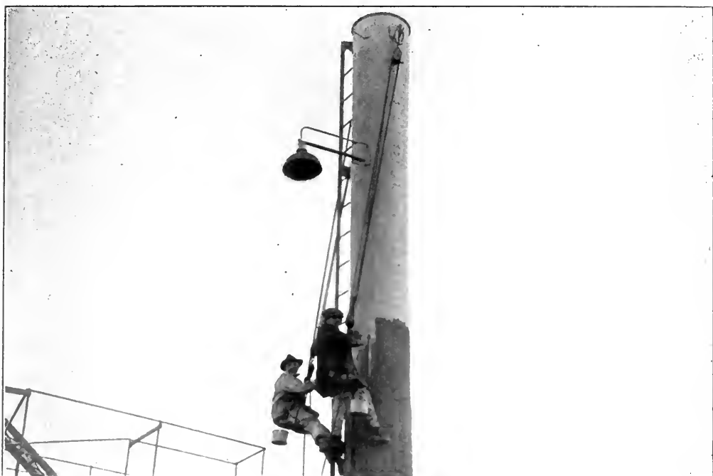
Painters at Work
