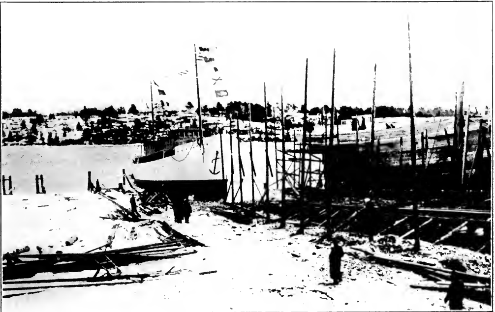
Ship just launched, with flags flying: launching ways showing at the right.
