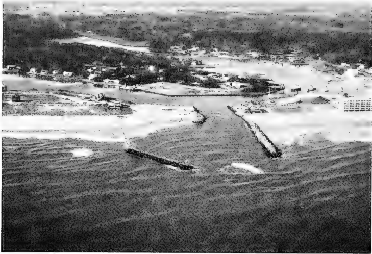
Figure 24. Weir jetty system at Rudee Inlet, Virginia Beach, Va. (Sand movement at this location is predominantly south to north (left to right in the photograph). Sand moves over the low weir section and is periodically pumped to nourish the recreation beaches north of the north jetty)
