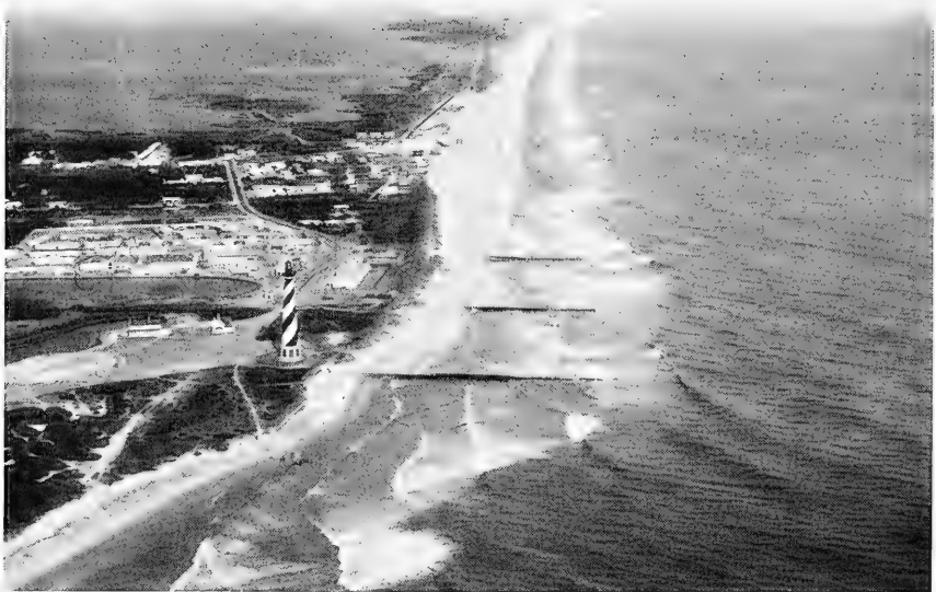
Figure 23. View toward north of groins near Cape Hatteras Lighthouse; Cape Hatteras Point is about 1 km south of the lighthouse (note the change in shoreline orientation at the groin system. Sand moving from north to south is partially trapped and held north of the groins. The beach to the south (bottom of photograph) consequently receives less sand than it loses, and erosion is accelerated)
