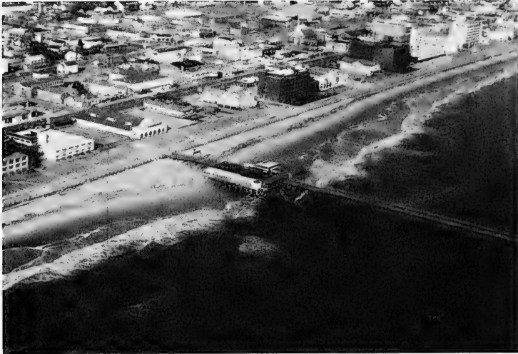
Figure 22. Recreational pier at Virginia Beach, Va., a typical fishing pier for the study area (note the shoreline bulge created at the pier by a decrease in the rate of sediment transport parallel to shore. The decrease probably occurred because the pier piles created a partial obstruction to shore-parallel flow and because the pier piles in the water dissipate some of the wave energy)
