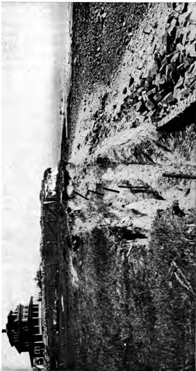
Wire fence undermined by wave attack and left hanging in mid-air. The road in front of the house has been completely cut away. Third Cliff, Scituate, Massachusetts.
