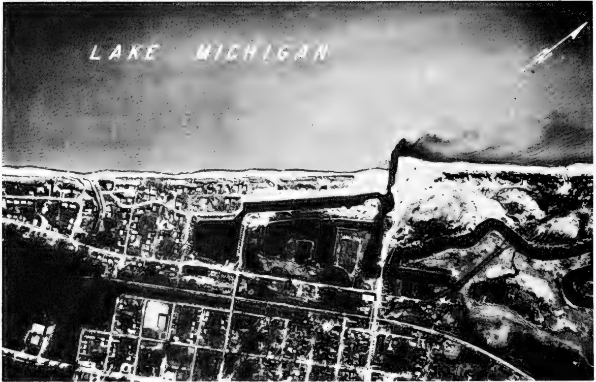
Figure 4-52. Transport directions at New Buffalo Harbor Jetty on Lake Michigan.
