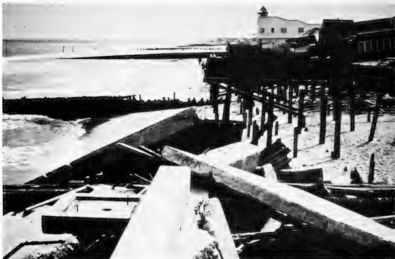
Figure 1-10. Damage after the 1962 storm, Rehoboth Beach, Delaware.
