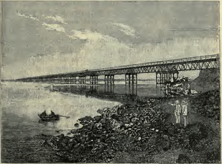
BIO-BIO-RIVER AND BRIDGE OF THE SOUTHERN RAILWAY.
