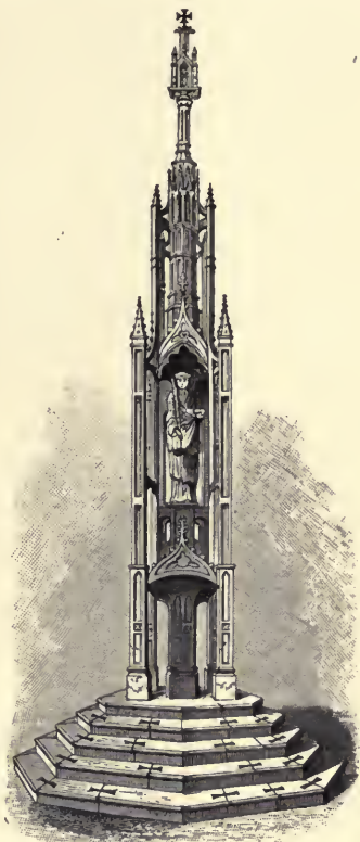
WINCHESTER MARKET CROSS. Built temp. Edward III.
