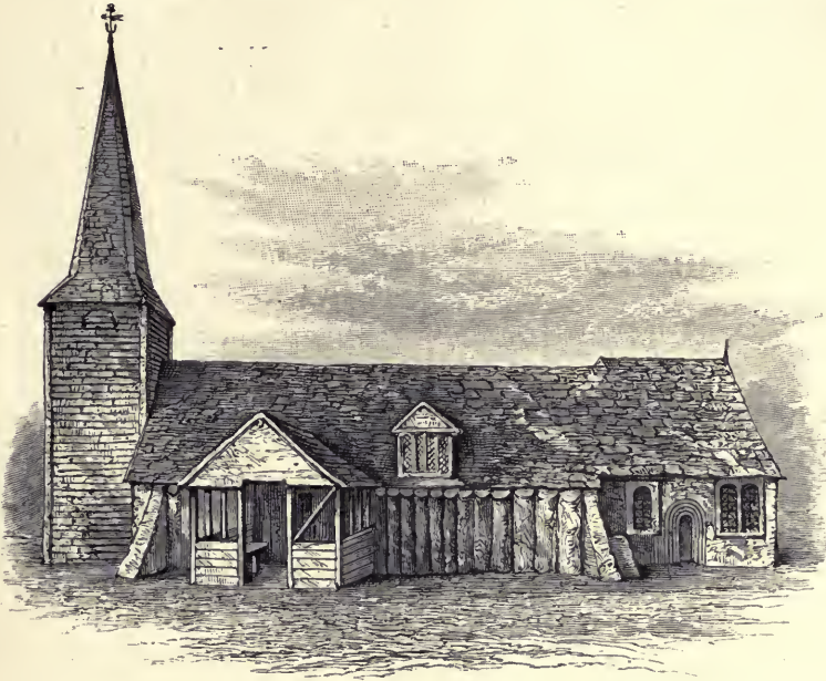
WOODEN CHURCH, GREENSTEAD, ESSEX, A.D. 1013 (AS IT WAS IN 1748). "Vetusta Monumenta."
