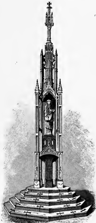
WINCHESTER MARKET CROSS. Built temp. Edward III.
