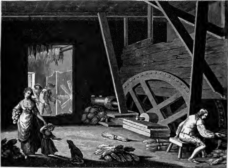
BREAKING AND SCUTCHING BY MACHINERY.
