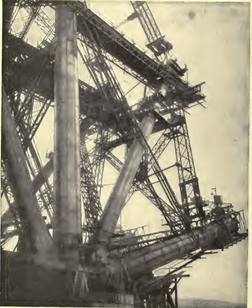
CONSTRUCTIONAL DETAIL OF THE FORTH BRIDGE
