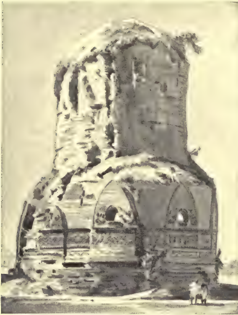
THE DHAMÊKH TOWER
