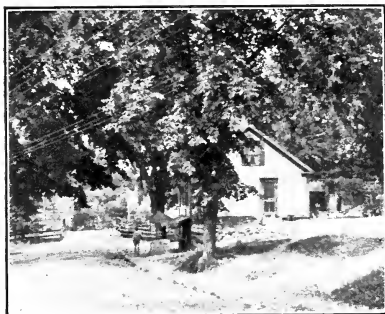
VIEW ACROSS THE BRIDGE THAT SPANS ABBOTT'S RUN
