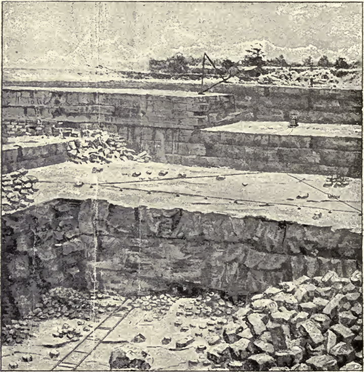
FIG. 65.—EXAMPLE OF SIMULTANEOUS BLASTING IN SERIES.
