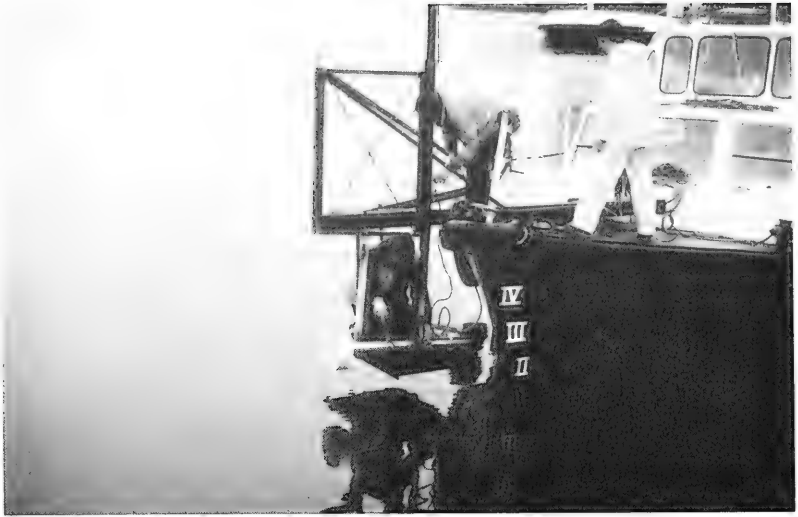
Figure 33. Side-scan sonar being attached to frame on work boat for precision survey of vertical wall structures in Quebec Harbor, Canada
