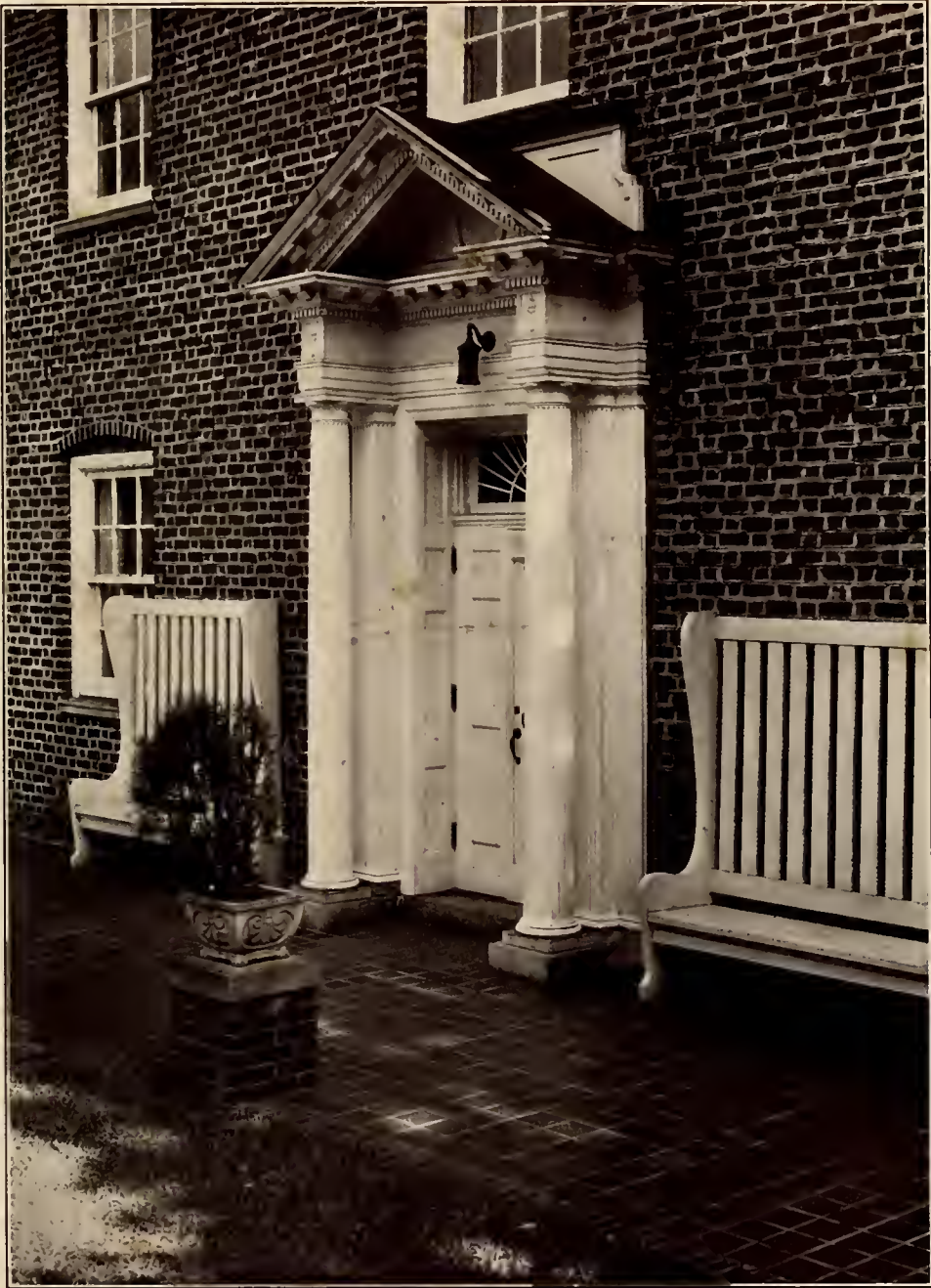
North Entrance to Alice Clewell Dormitory
