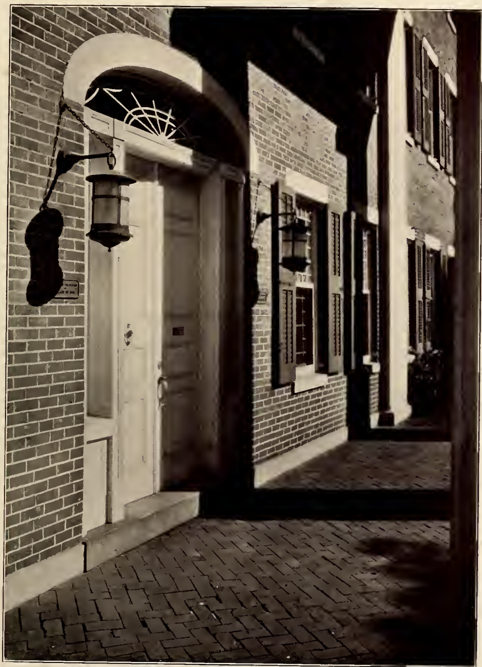
Entrance to Main Hall
