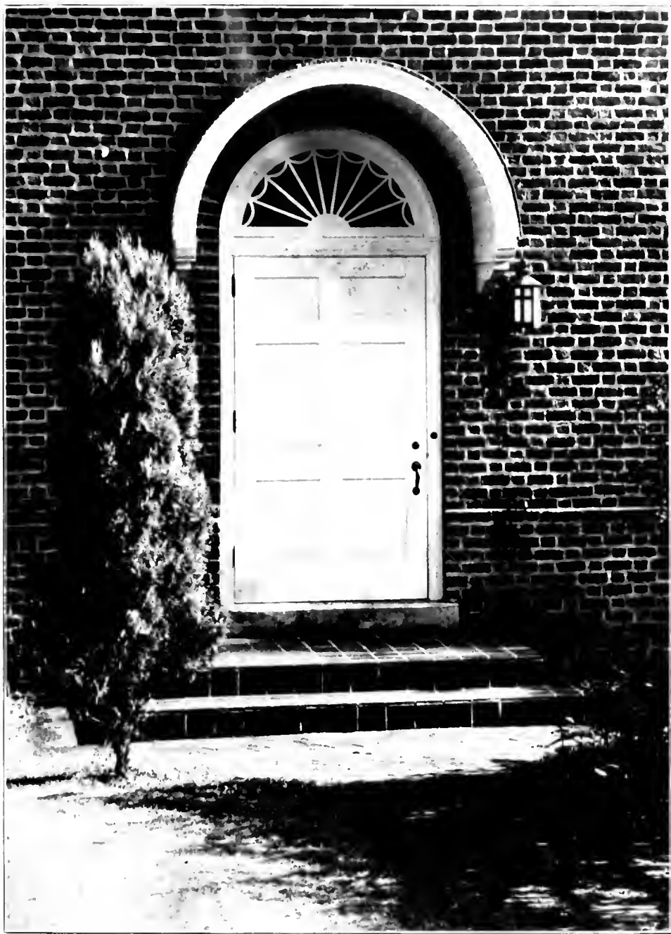
Entrance to Bahnsen Infirmary
