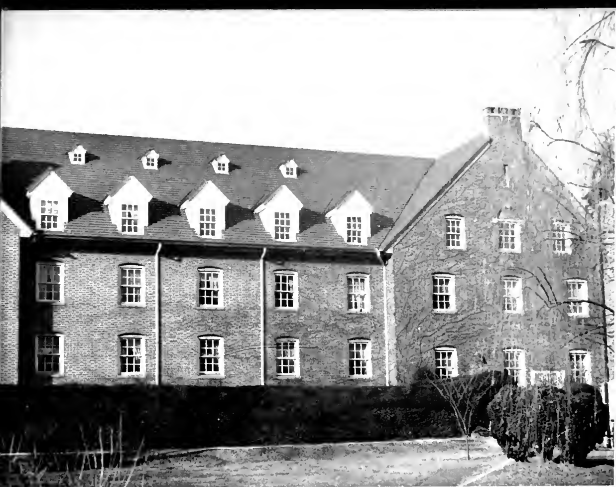
East View of Alice Clewell Building
