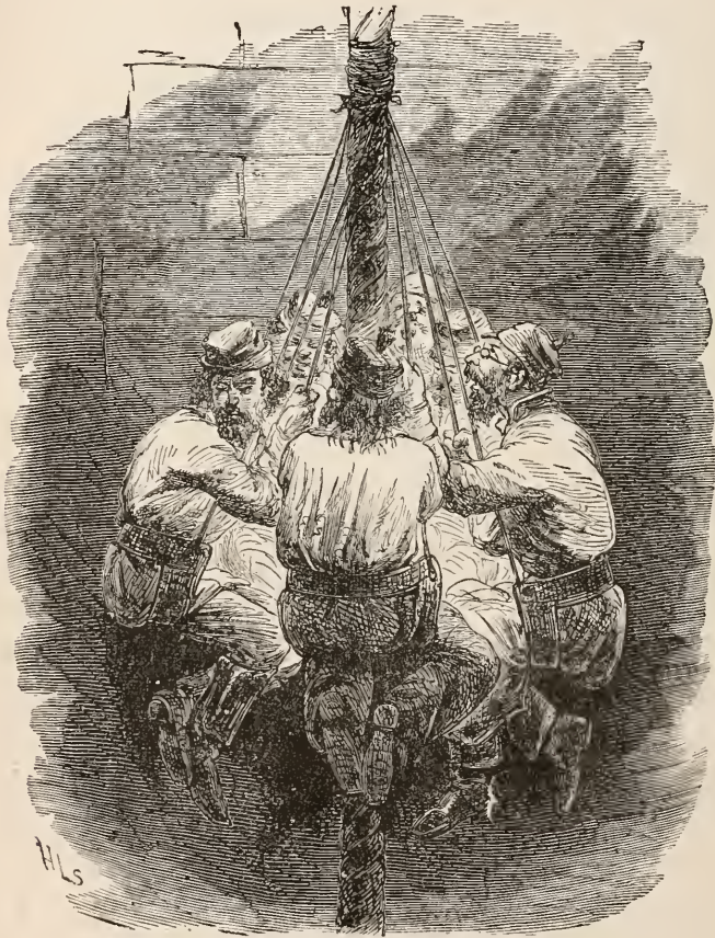
DOWN THE SHAFT.
