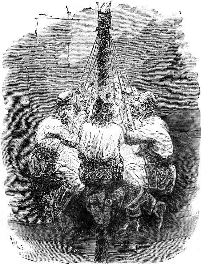
DOWN THE SHAFT.
