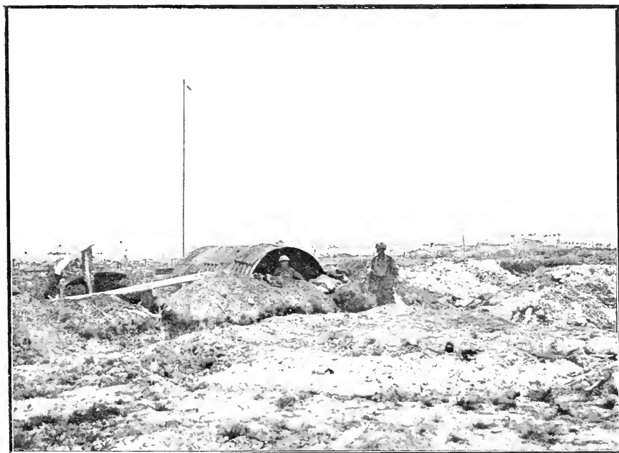
A forward Wireless Station.
