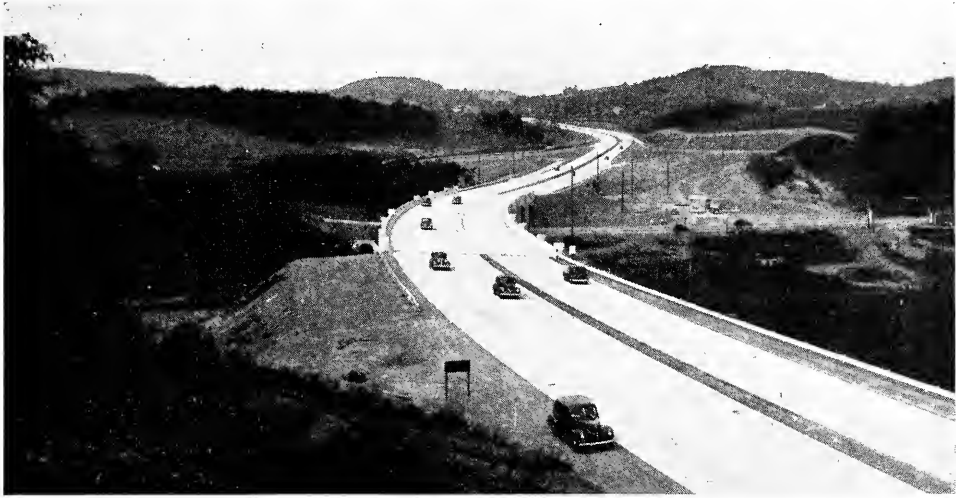
Safety engineers laid out the moderate curves so that any of them can be taken at 75 miles per hour without strain.
