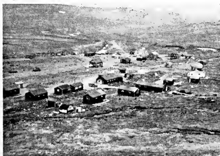
Typical Mining Camp. Goodnews Bay Mining Co. Camp, Platinum, Alaska. Note treeless landscape, tundra covered.
