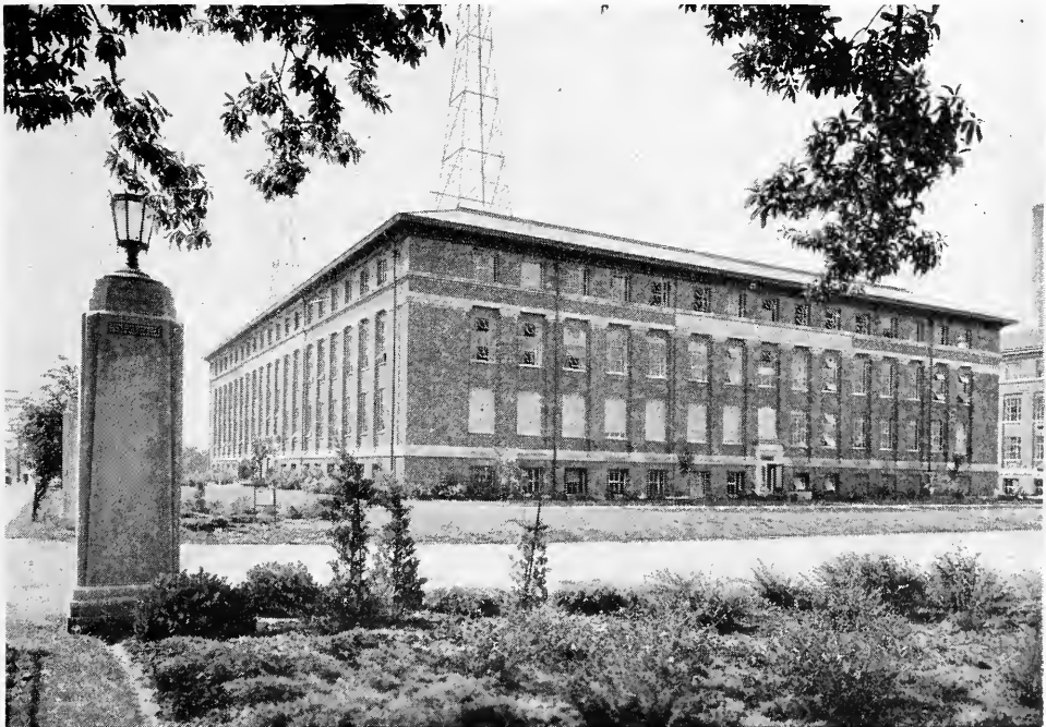
ELECTRICAL ENGINEERING BUILDING
