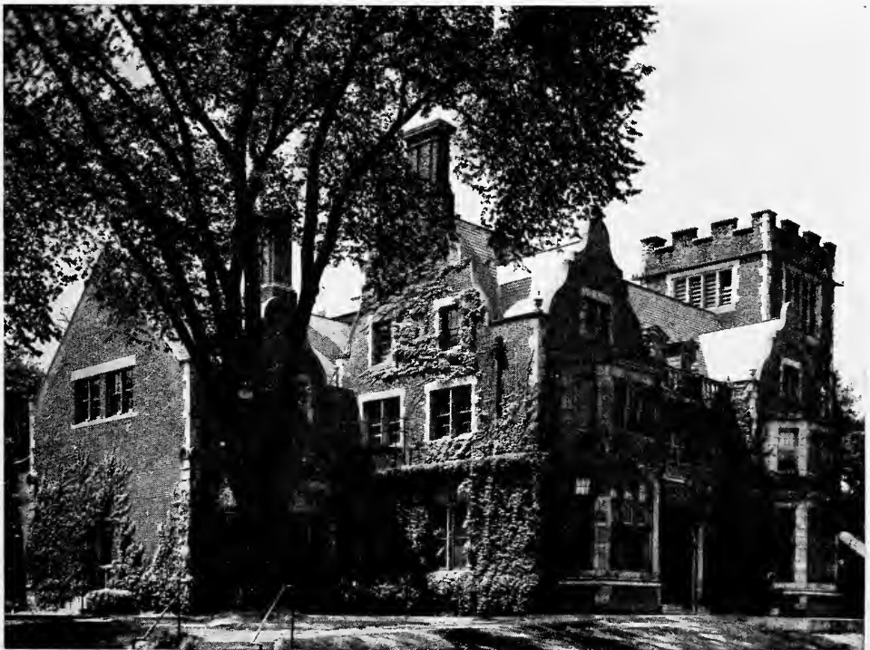
Coxe Hall, the main administration building.
