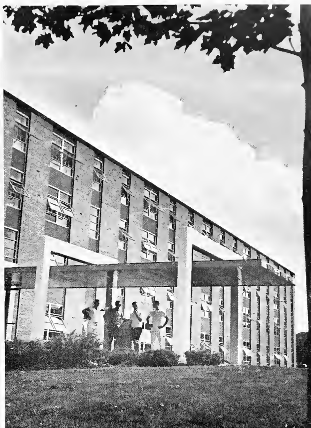
Bertha G. Beull Residence Hall at Eastern Michigan
