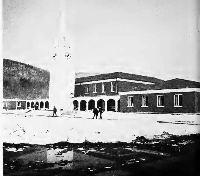
Library at Quinnipiac College, built to accommodate 100,000 volumes
