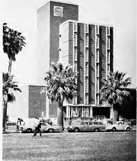
University of Arizona Administration Building
