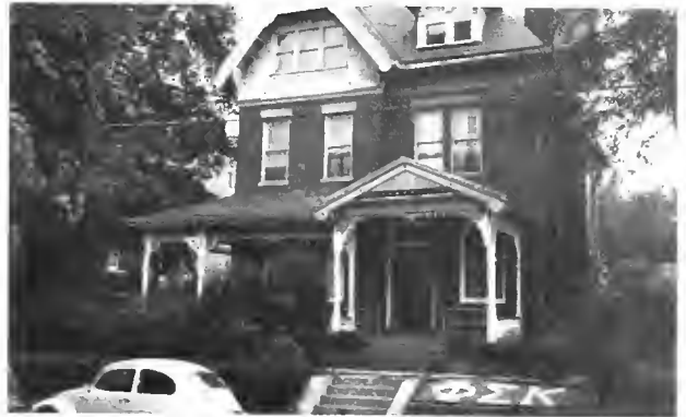
Above is a picture of the old house which has been given up pending the procurement of a new house.
