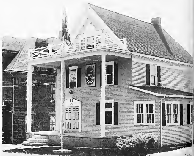
Theta Pentaton House after renovation
