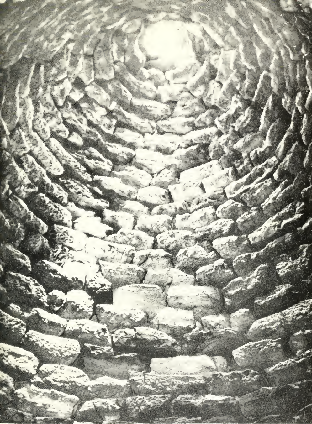
[32] Looking up through the interior of a nuraghe. These austere buildings provided Sardinian chieftains with living quarters and their warriors with an almost impregnable stronghold.
