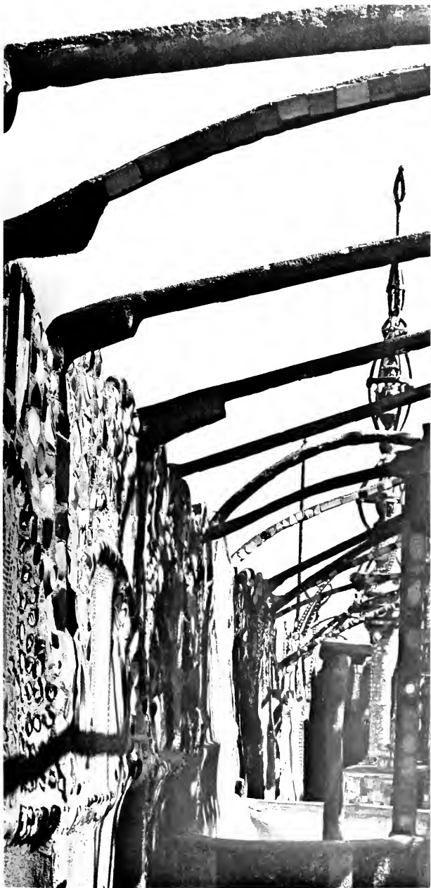
Inside the North wall looking East
