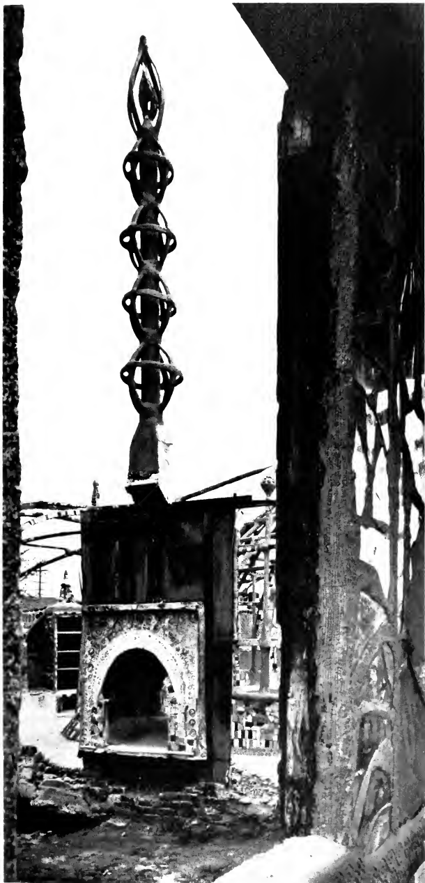
Inside the South entrance looking Northeast through what was once a window of Simon Rodia's house. All that remains is this wall and the fireplace.
