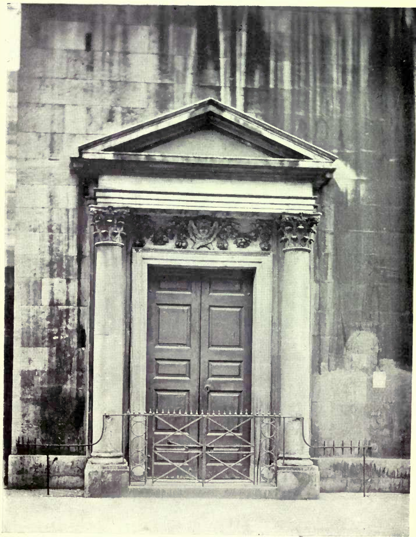
PLATE 50.—DOORWAY, ST. MARGARET'S, LOTHBURY
