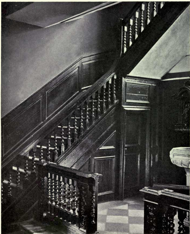
PLATE 47.—STAIRCASE AT ST. MARY ABCHURCH
