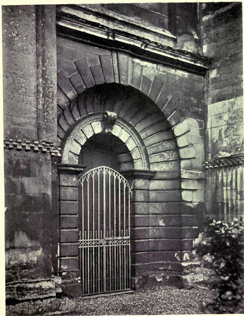
PLATE 4.—DOORWAY, NORTH TRANSEPT, ELY CATHEDRAL
