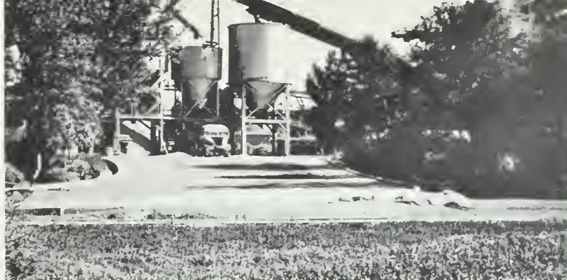
Figure 74 — Dominant focal points of structures can be softened and masked with transition planting
