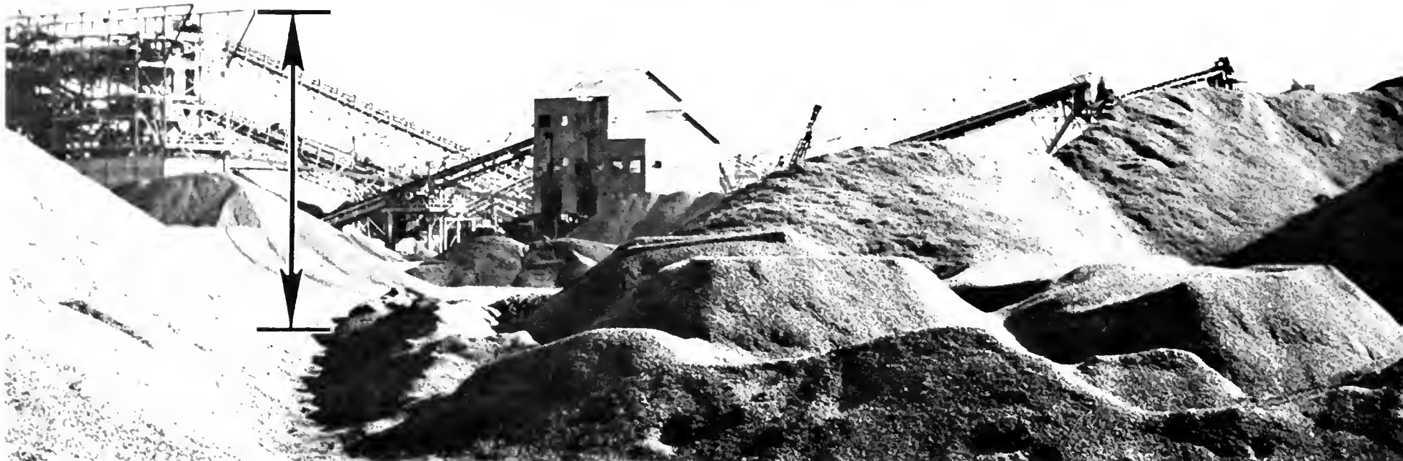
Figure 68 – Multipurpose land forms – stockpile forms provide effective screens for views upon the processing plant (Image areas 1, 2 and 3)
