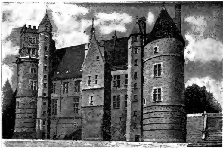
Facade d. Hauses zu Bourges.
