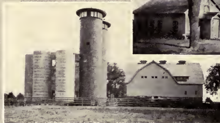
Animal Husbandry Silos
