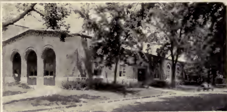
Gas Engine Annex
