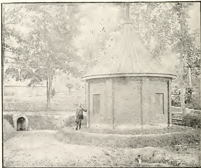
INSTITUTE SPRING AND PUMP HOUSE.
