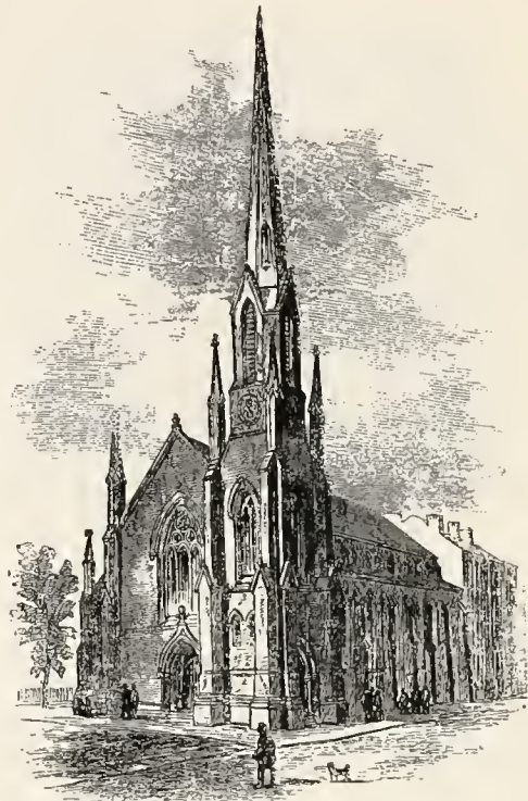
THIRTEENTH CONGREGATIONAL CHURCH. HARRISON AVENUE, CORNER OF BEACH STREET.
