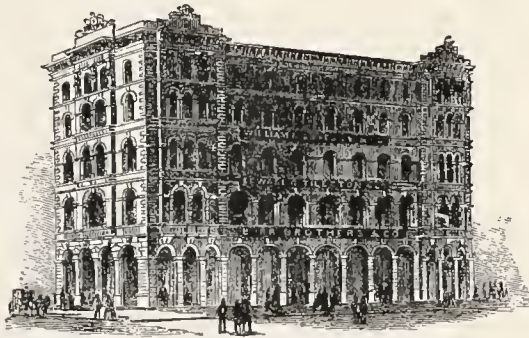
View of Building 74 and 76 Franklin Street.
