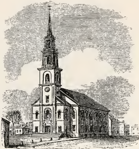
HOLLIS STREET CHURCH. HOLLIS STREET.
