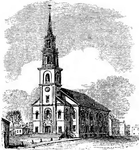
HOLLIS STREET CHURCH. HOLLIS STREET.
