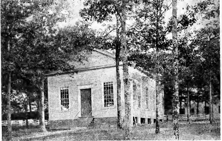
Asheboro Presbyterian Church on Worth Street. Organized 1850; building erected in 1851-1852.
