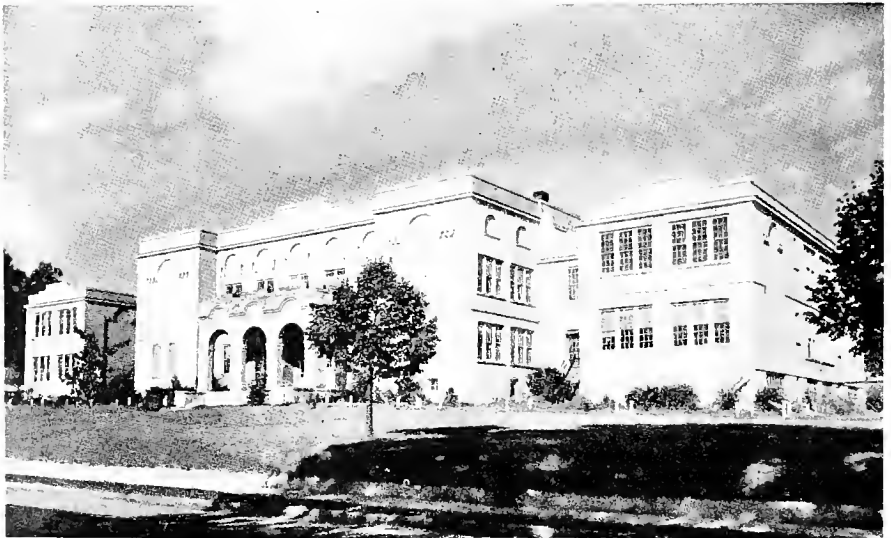
Fayetteville Street School after the wings were added 1923-1926. This property was sold in 1969 and the school was torn down, thus ending more than a hundred years of its use for school purposes.
