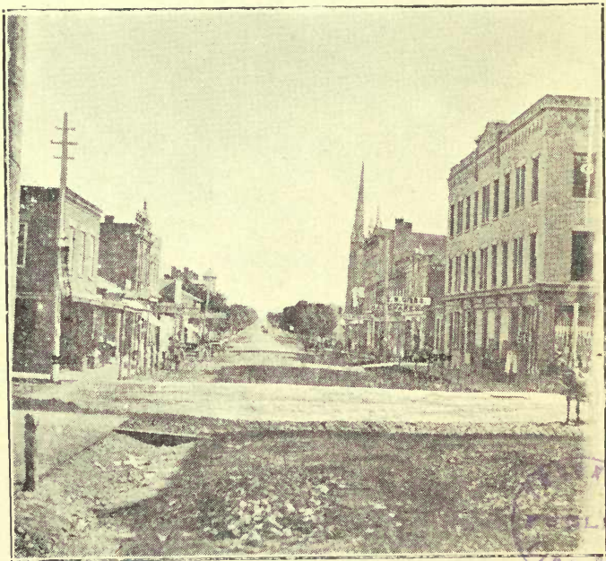
COR. KING AND SIMCOE—1871—LOOKING SOUTH [Photo by W. H. Kirby]
