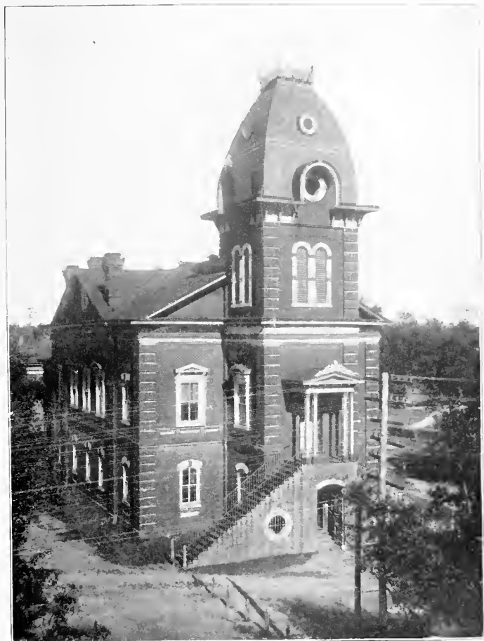
MARLBORO COURTHOUSE, ERECTED A. D. 1885.
