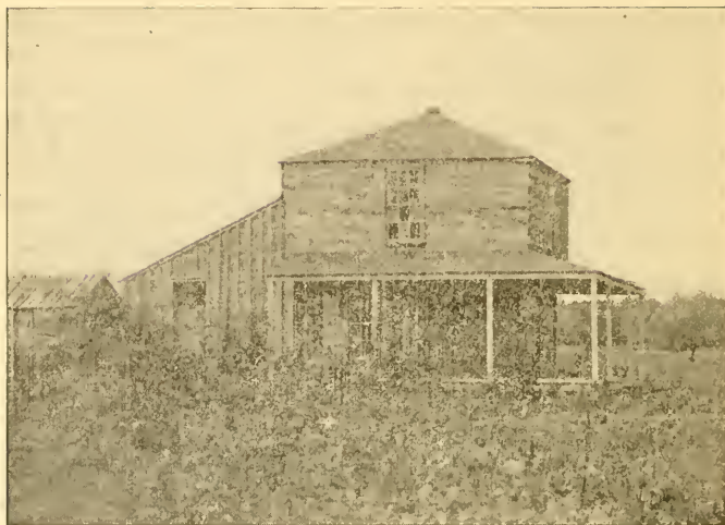
THE REMAINING BLOCK HOUSE,
