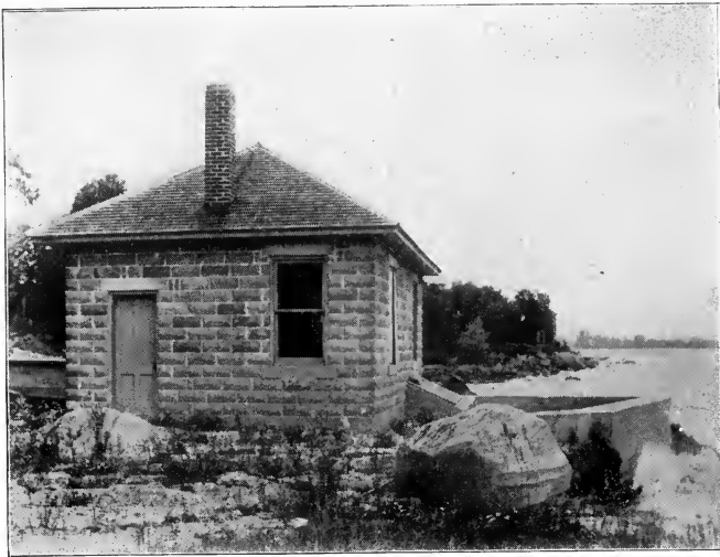
Waterworks Pumping Station
