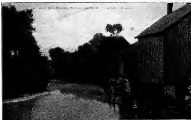
West Side Pumping Station
