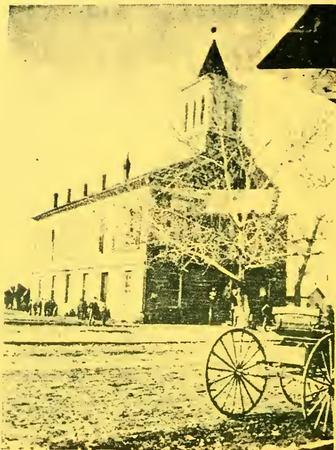
COURT HOUSE OF JACKSON COUNTY, in which the trial took place
