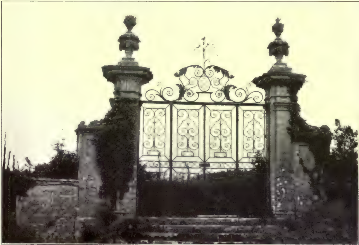
PLATE 170. Gate from garden to farm, Château de Brécy, near Bayeux
