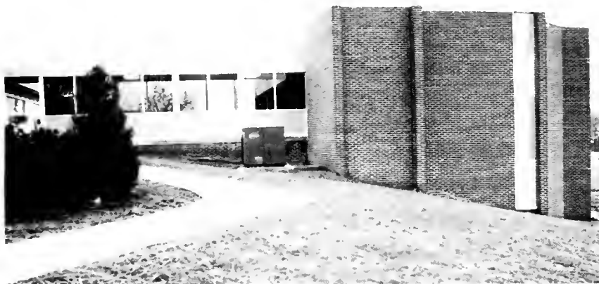
This is the new addition to the Spalding Elementary School, with its four classrooms and four restrooms. It houses the seventh and eighth grades which have two sections each with a total of 120 pupils. On the left is the connecting passage between the old and new parts of the building.
