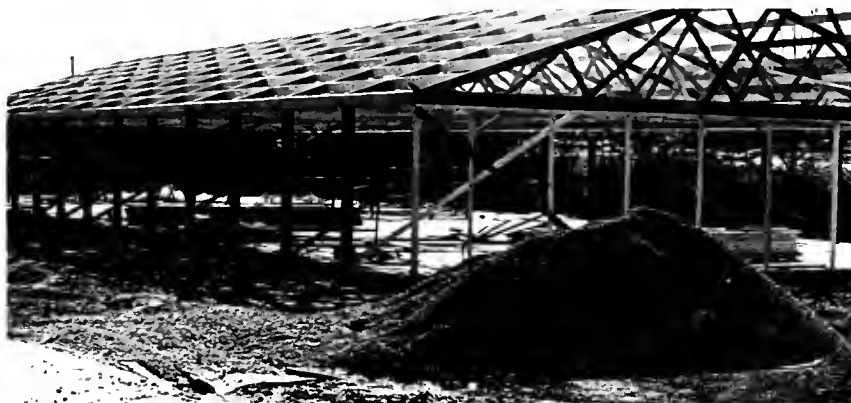
The new greenhouse in which hydroponic tomatoes hopefully will be produced commercially.
