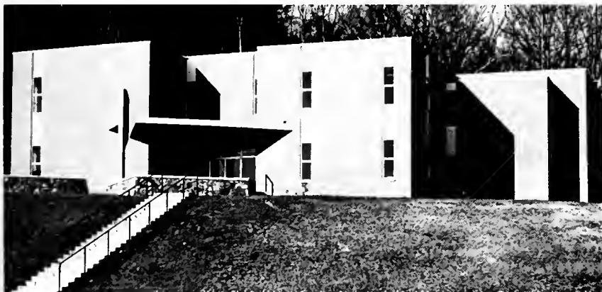
Front view of the new Home Economics Building.
