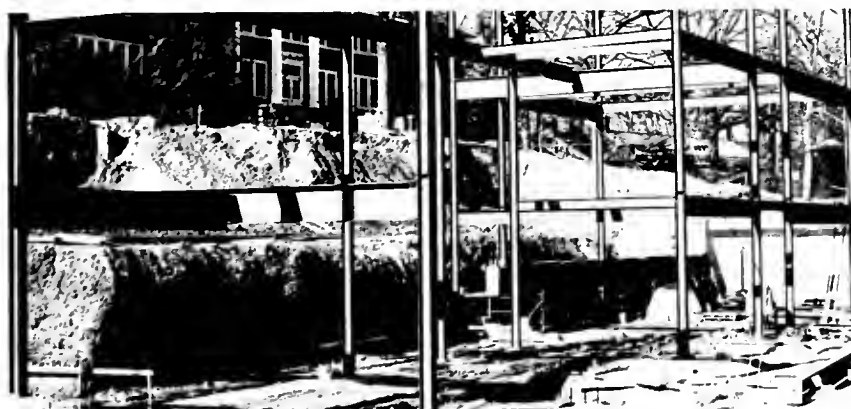
This picture shows the progress on the new cafeteria building which is being erected on the site of the former cafeteria just back of Wright Hall. The old tabernacle houses the food service department until the new one is completed.
